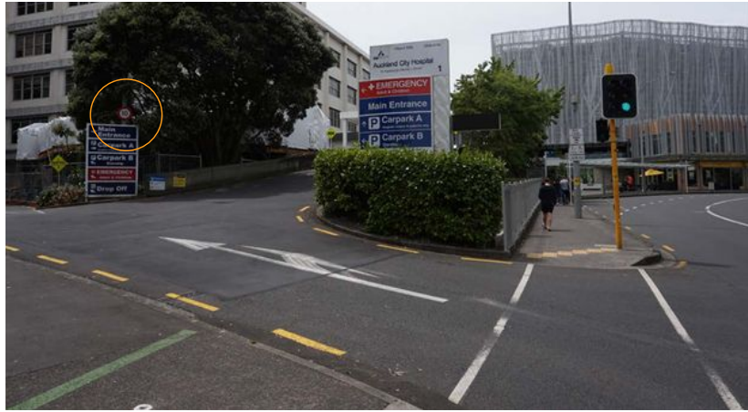
Ill placed speed zone indications
