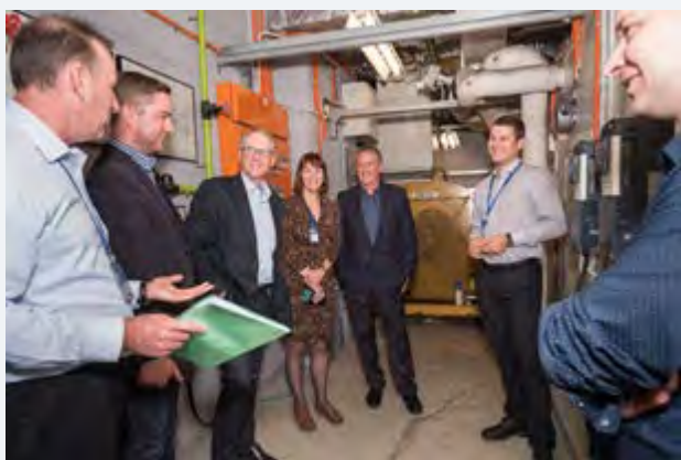
Reviewing the oncology building's HVAC plan which has been optimised to save energy through the EECA collaboration
